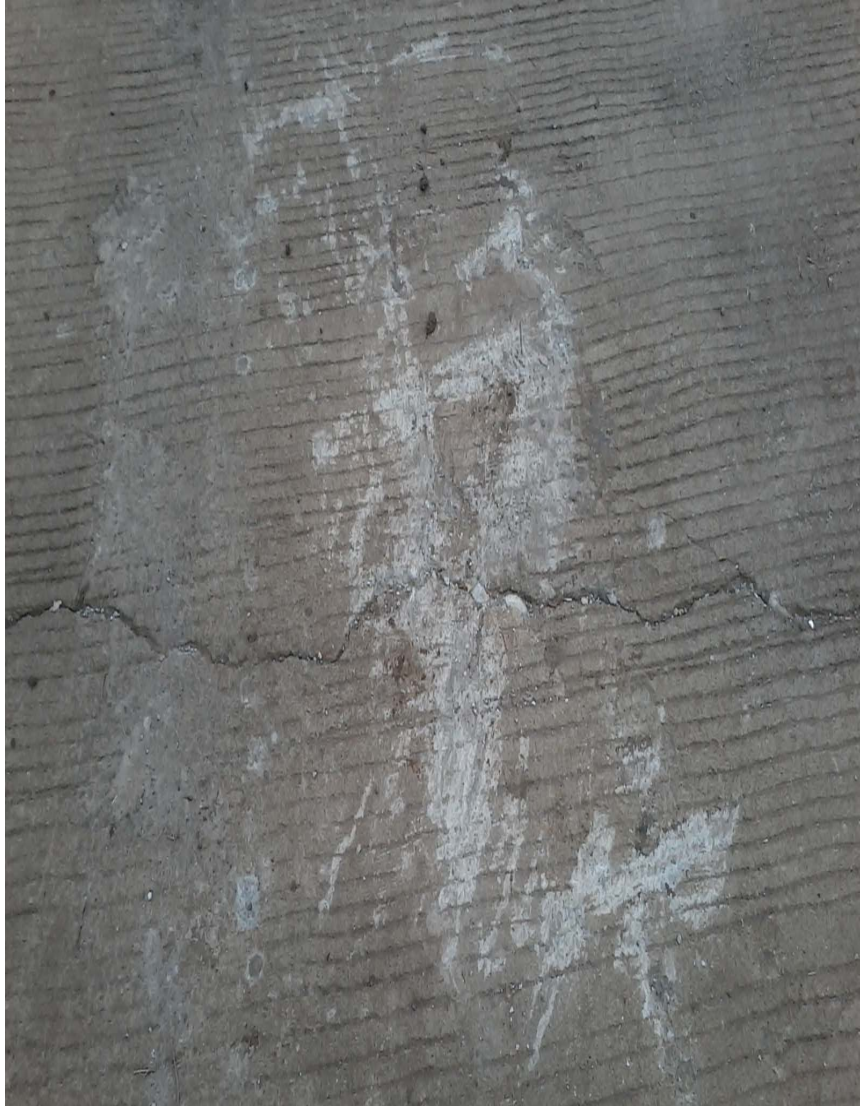
CONCRETING OF ROAD ALONG SITIO TIMANO, BRGY. BINATON, DIGOS CITY
